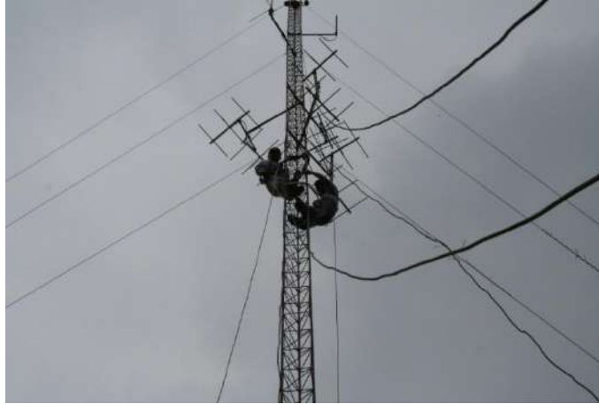
Figure 2. Installation of telecommunications node
