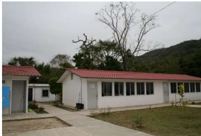
Figure 3. Interconnected classrooms at the Indigenous University of San Luis Potosi in Matlapa.
